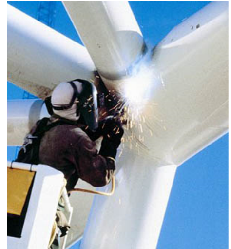
Figure 1. Wearing dark clothing during a weld will protect you from the arc's harmful rays.
