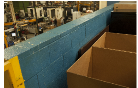
Figure 1: Guard walls help to prevent falls.
