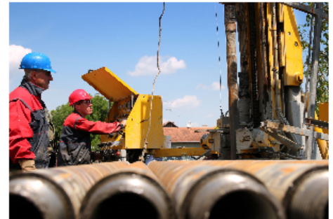
Figure 2: Oil and gas drilling is a high-hazard industry.
