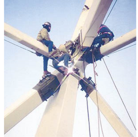
Figure 1. A welder performing shielded metal arc welding on site.
