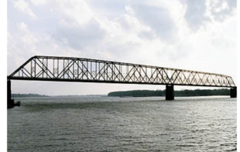
Figure 1. The metals used to build this bridge were welded together.
