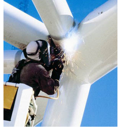
Figure 1. Shielded metal arc welding performed on site.
