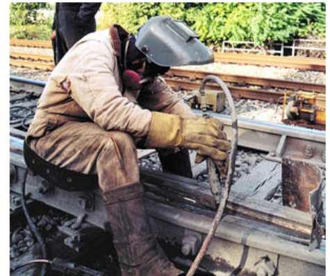
Figure 2. Chipping slag from the welded metal.
