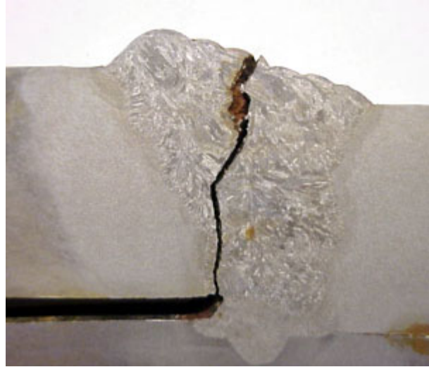
Figure 1. Small cracks and a lack of toughness led to failure of the weld.
