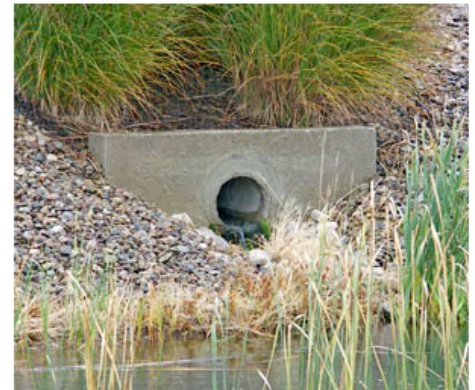
Figure 2. A sewer is considered a limited-access confined space.
