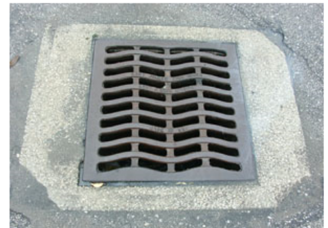
Figure 2. Sewers and drains are considered confined spaces.
