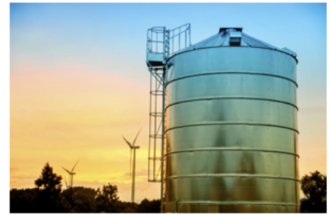
Figure 1. A confined space that contains an engulfment hazard, such as the grain in a silo, requires a permit for entry.
