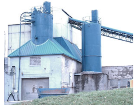
Figure 2. These industrial silos contain powdered materials for making concrete blocks.
